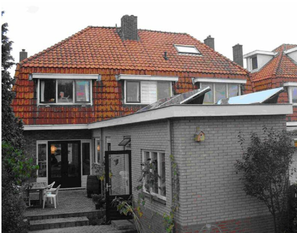
Solar system of 560 Wp on an extension from the 1980s of a typical Dutch semi-detached house from the 1930s.
